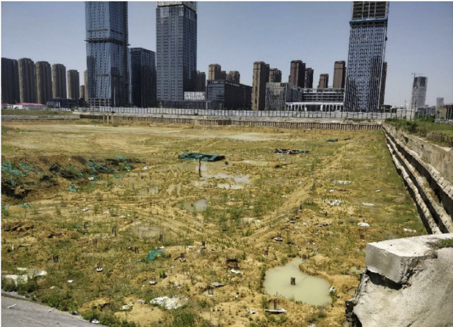
Fig. 2. Status of foundation pit.
