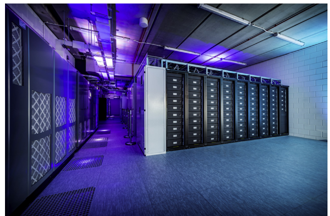
Fig. 2. Racks with part of the 2.8MWh energy storage system at the “Johan Cruyff Arena”. [Photo courtesy of Eaton].
